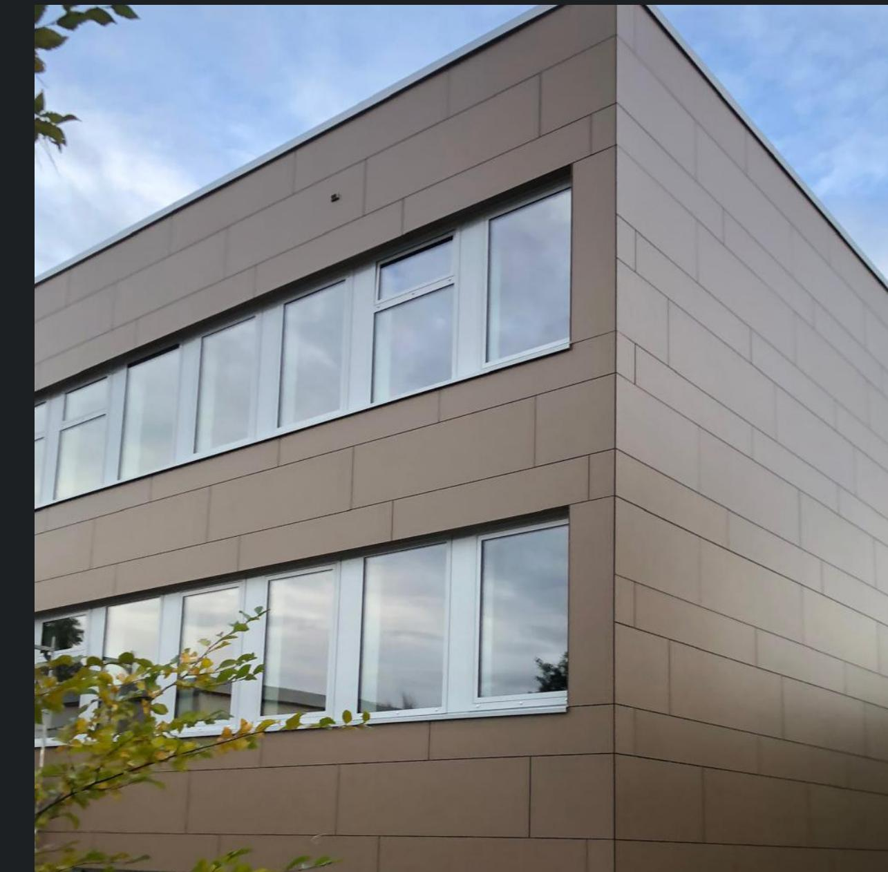
These façades consist of two separate layers of cladding elements with an air gap in between. This design ensures effective ventilation and provides additional protection against environmental factors.
