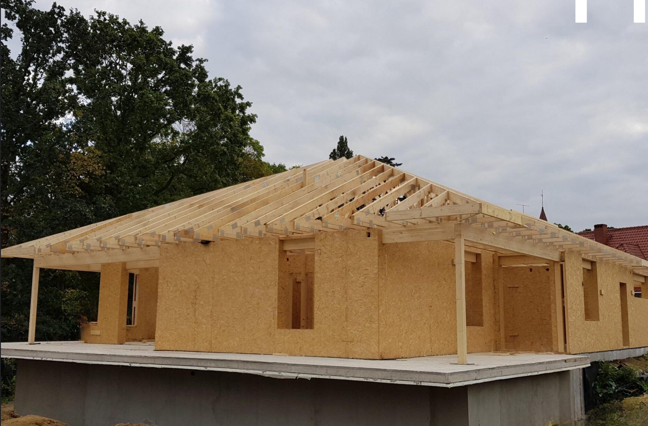
We specialize in constructing houses using timber frame technology, incorporating KVH-C24 structural wood, which guarantees durability and stability. Our projects combine modern technologies with the natural beauty of wood, providing comfort and energy efficiency.
