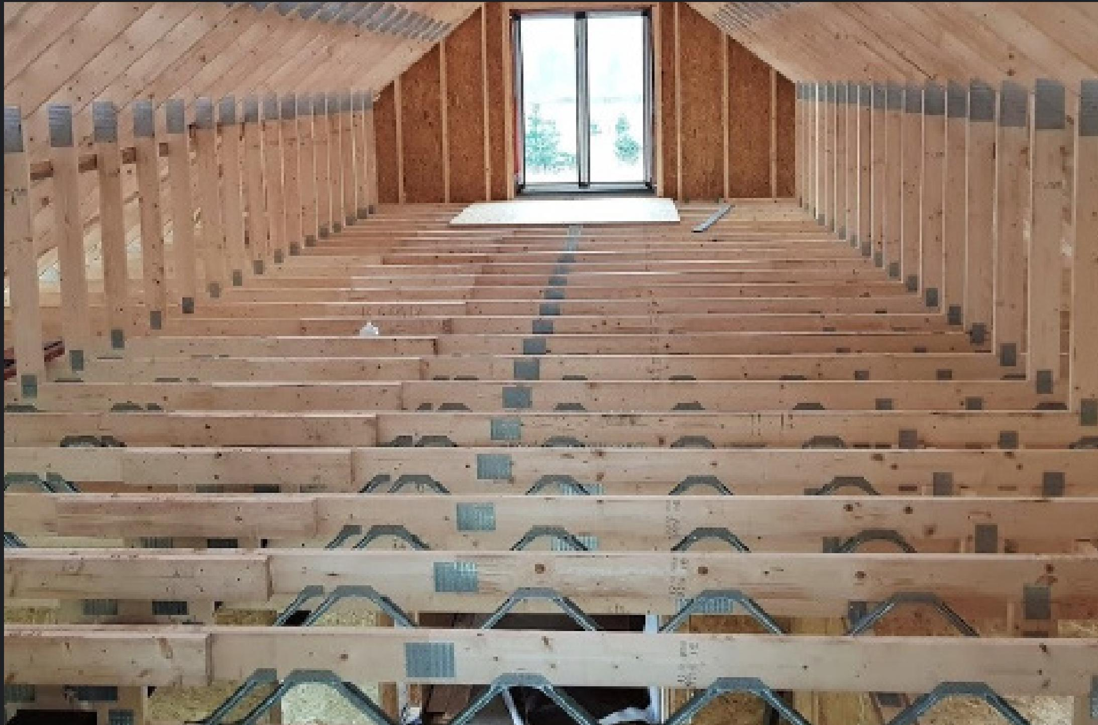
Timber-steel Posi-Joist beams combine lightness and strength with easy installation and processing. Their popularity has grown significantly in Western Europe and is now rapidly increasing in Poland.
