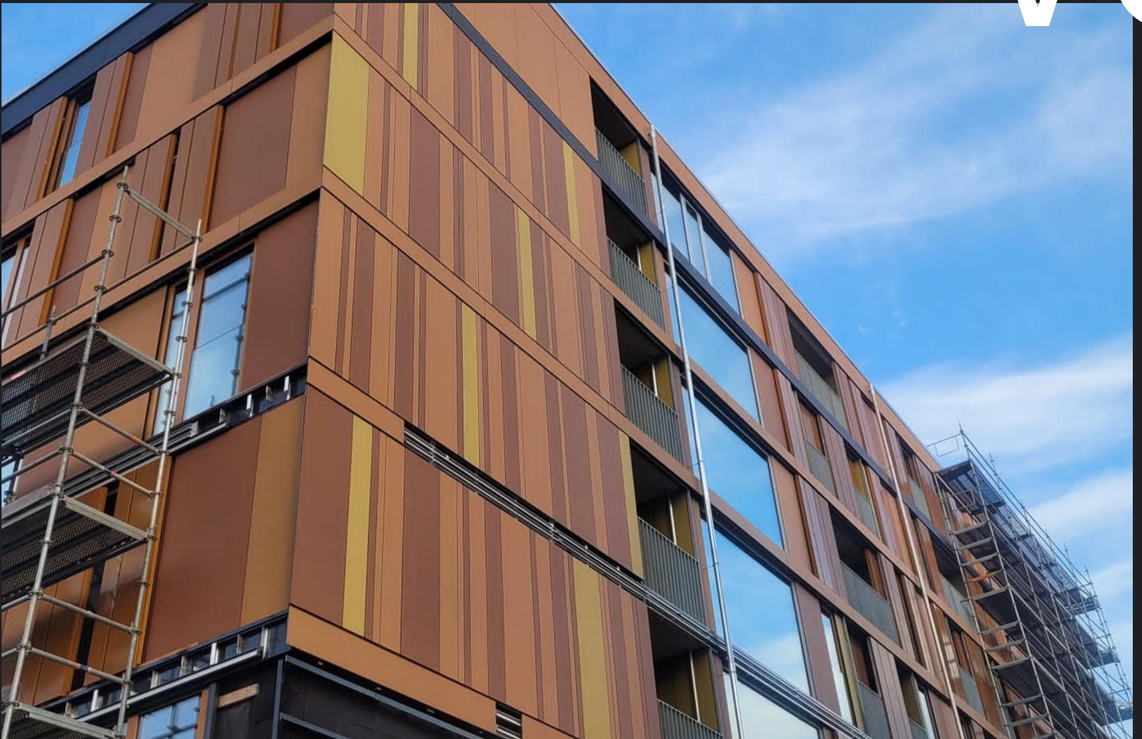
Ventilated façades are a type of cladding system where an air gap is created between the external cladding and the supporting wall structure. This gap enables controlled air circulation behind the façade.
