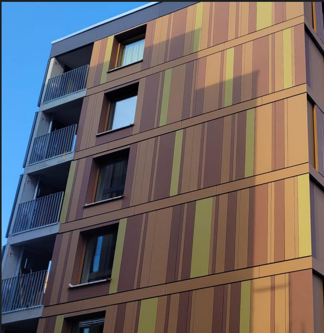
In this type of façade, the cladding elements are not directly attached to the supporting structure but are mounted using a separate frame. This creates an air cavity that allows for air circulation.
