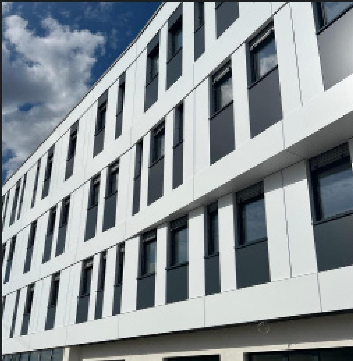
This façade type features an external layer of cladding that is attached to the supporting wall via a structural frame. Behind this cladding layer, an air gap ensures proper ventilation.
